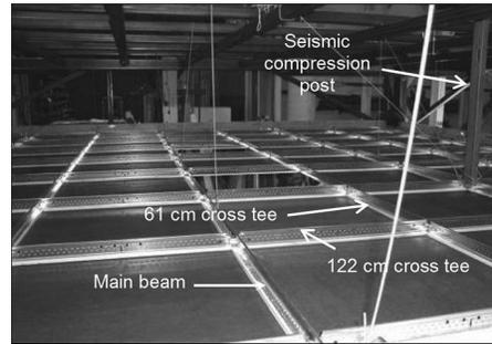
**Figure 2.** Suspension grid components.
